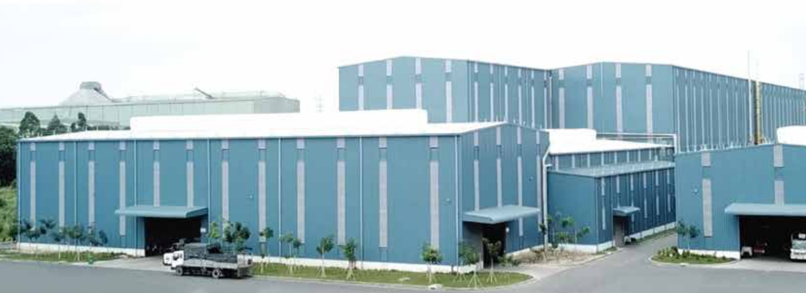
Pomina Flat Steel Mill, Ba Ria - Vung Tau Province
