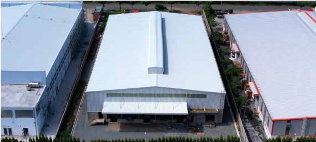
Long An Postal Transport Operations Center
