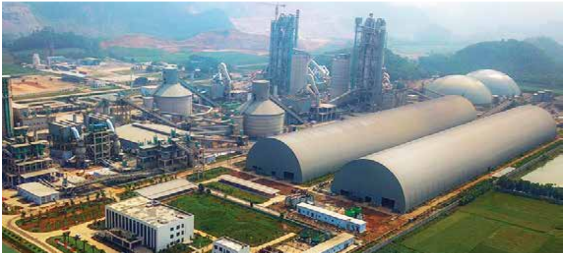
Long Son Cement Factory, Thanh Hoa Province
