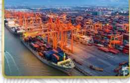
CẢNG NƯỚC SÂU DEEP-WATER SEAPORT
